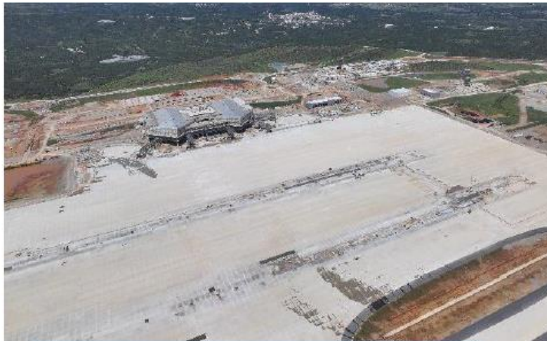
Apron Pavement Works
