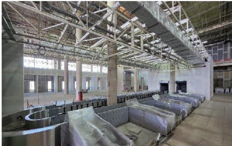
Terminal Building: Baggage Handling works at Check-in Hall
