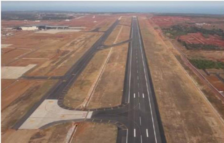
Runway and Cross Taxiway
