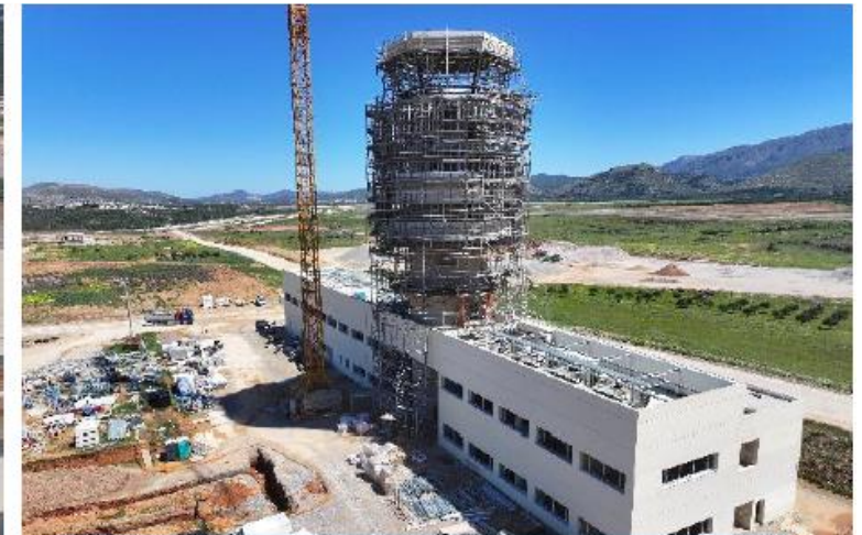
Control Tower Works
